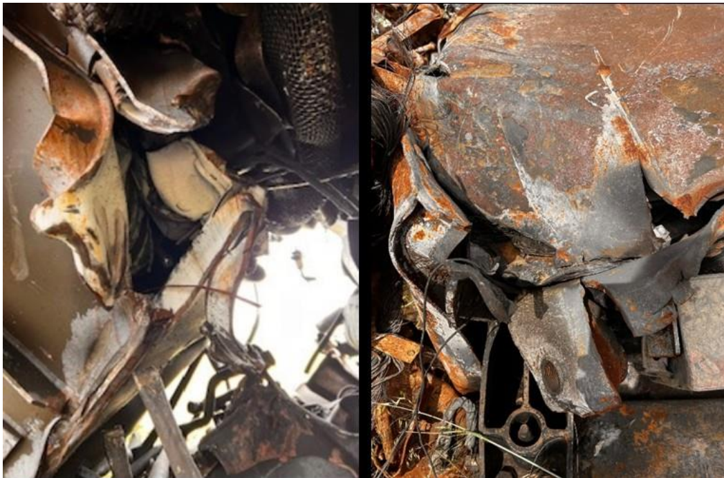
Figure 67. Large cracks of the transformer still attached under the 120-022 locomotive (Left). Bumps, folds, rips and large cracks of remaining locomotive transformer 120-023 (right), see also Figure 61.
