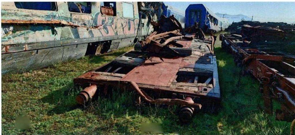
Figure 80. Position 4) nr 2 platform carrying steel plates, lost bogies from derailment but very slightly damaged, no signs of heavy crash.
